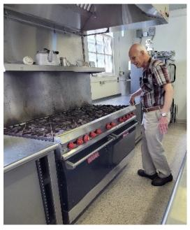
Ron G. took the stove's measurements. It is 6 feet wide and 30 inches deep with a height of 58 inches with its back piece of stainless steel. It is commercial grade and weighs 750 pounds. It is a Vulcan, but the model number, probably on the back of the stove, isn't available. The big range hood was required by the County and must be inspected every 10 years, Ron notes. To operate the stove, there is a gas valve on the wall and a pilot light that is lit manually.
